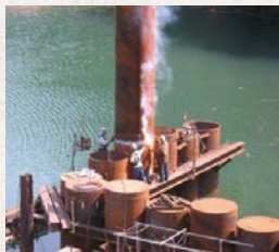
鋼管矢板継手溶接状況 ▶
